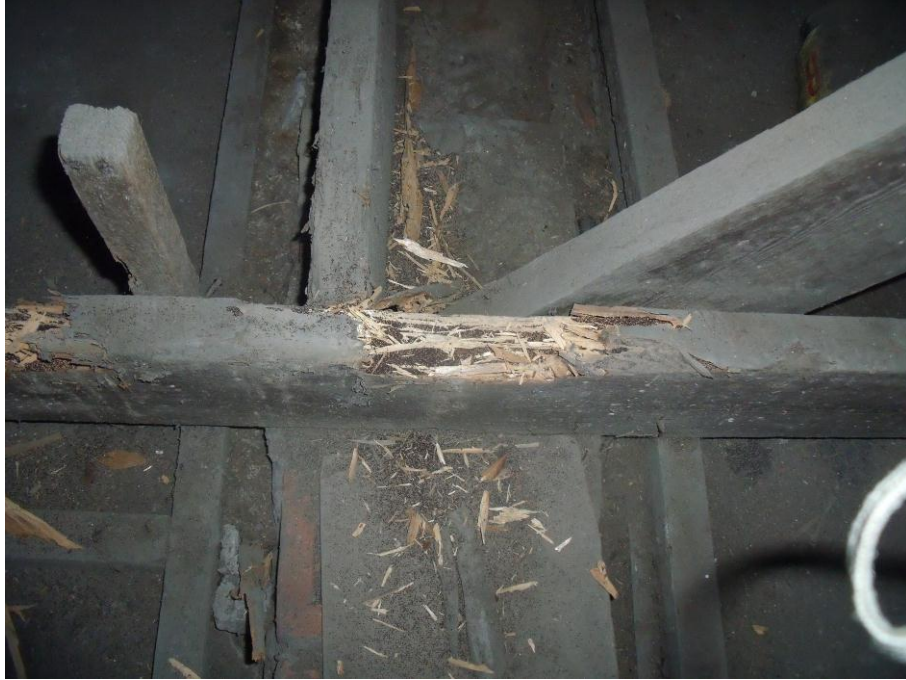
Figure 6- Wood borer damage on truss
