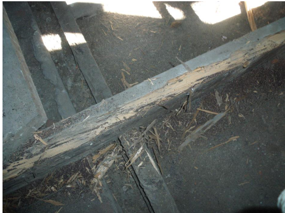
Figure 6- Wood borer damage on truss
