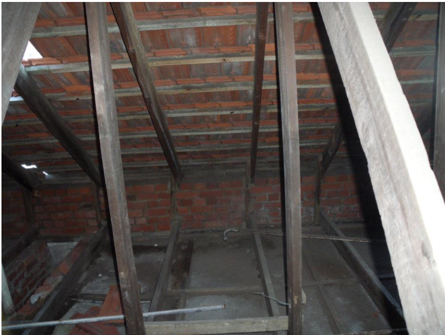
Figure 4- Buckling Webs
