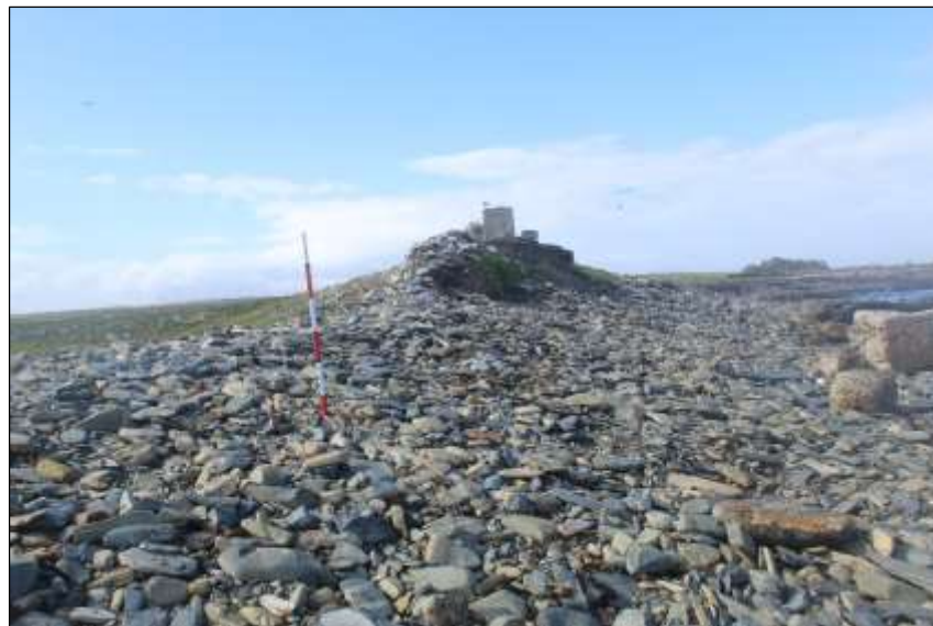
Figure 3: Collapsed section of the main wall, will be rehabilitated by anastylosis
