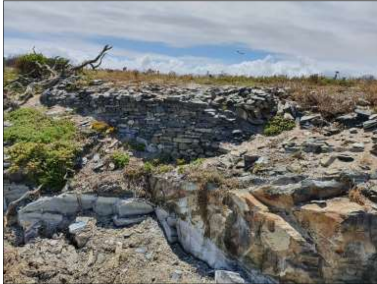
Figure 9: This revetment wall is of refined workmanship.
