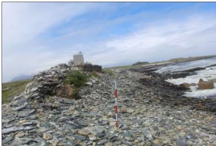
Figure 5: Scree of collapse facing the sea. It is possible that there was no wall on the seaside of the dyke.
