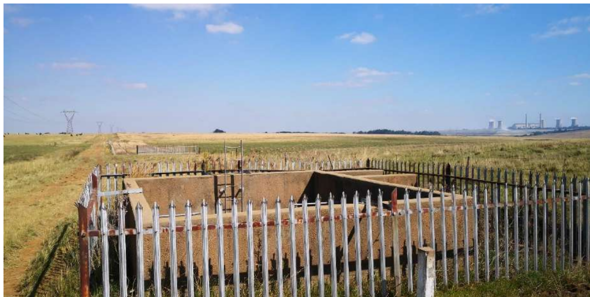
Mine infrastructure, leading to hardened surfaces, increased AIPs and changes to the natural hydrology, geomorphology and vegetation.
