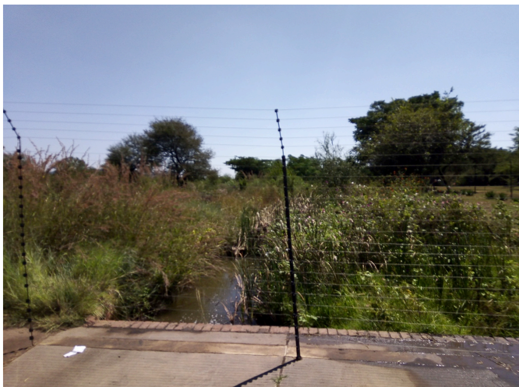
Photo 4: Low level bridge and road crossing over stream (Tsamma St)
