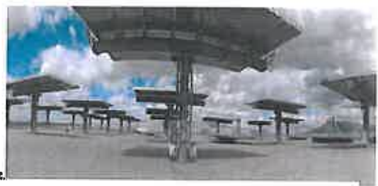
In stow: >26 mah. > 18 sec. Out of stow : <26 mah. >300 sec. Figure 4: Storm Stow position
