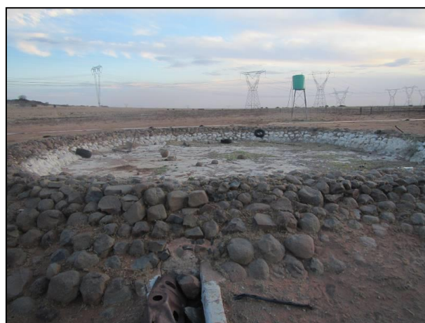
Figure 8.33: Stone dam a Waypoint 929.
