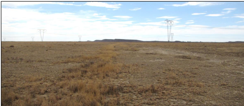
Figure 8.28: View towards the south across the eastern part of the project site
