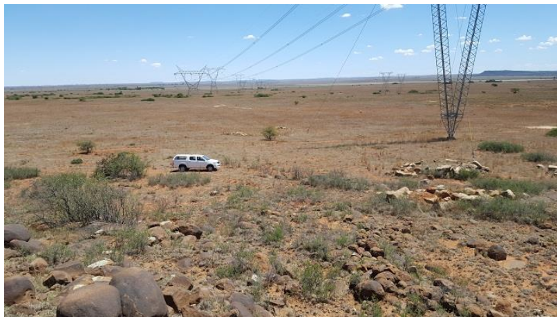
Figure 8.14: Photograph showing general site conditions. Note dolerite outcrop in foreground. Dolerite occurs at shallow depth below Hutton soils in the eastern part of the site.
