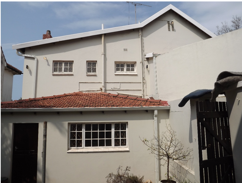
NORTH WEST ELEVATION FROM GARAGES
