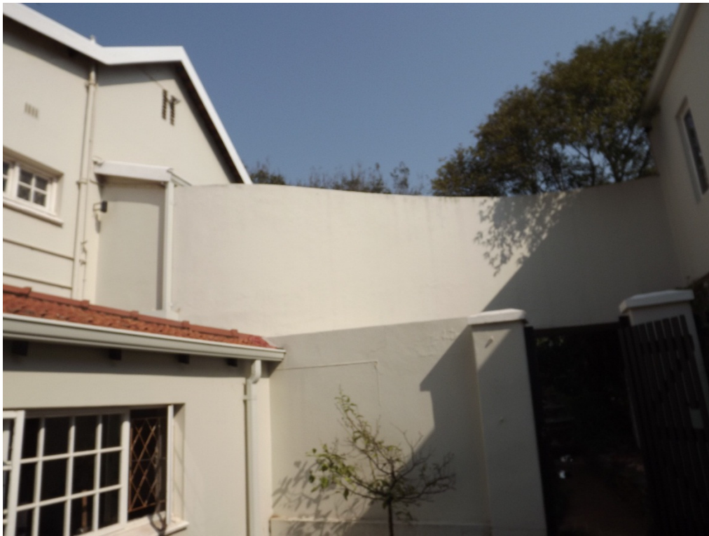
SOUTH EAST VIEW OF RAMP TO BE DEMOLISHED
