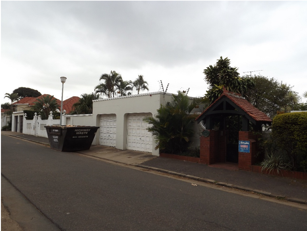
NORTH WEST ELEVATION FROM STREET
