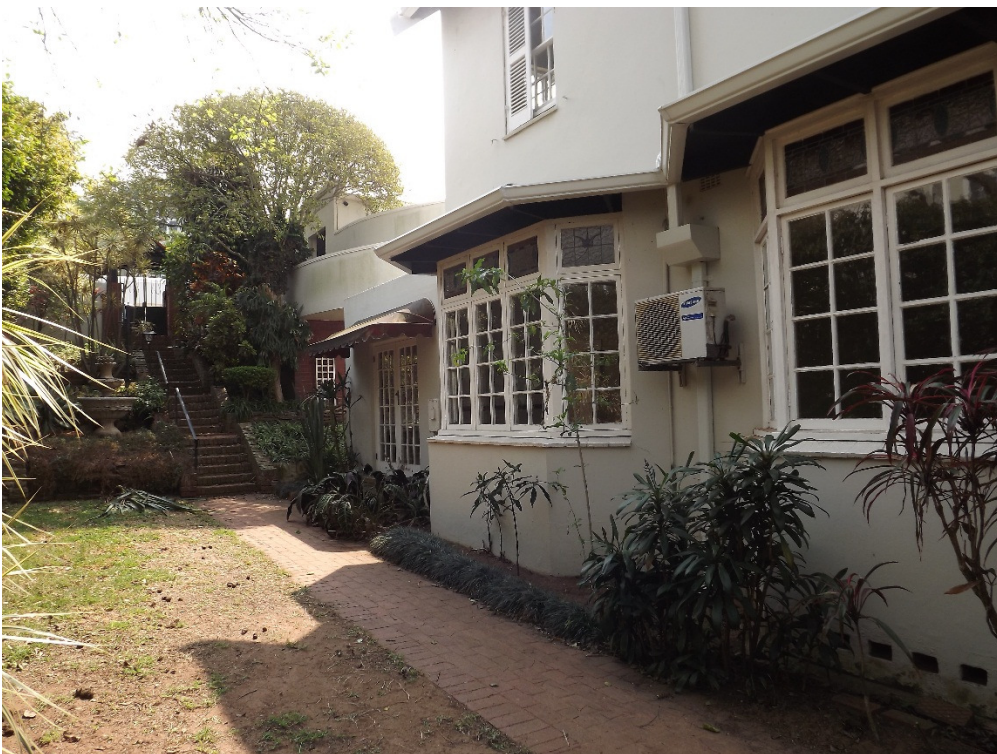
SOUTH WEST ELEVATION WINDOWS
