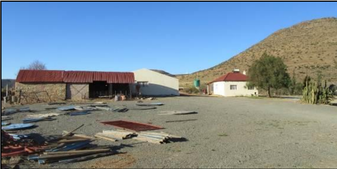
Photograph 3.12: Guest accommodation on The Dairy, with extensions in progress. A Noupoort WEF turbine is just visible between the buildings
