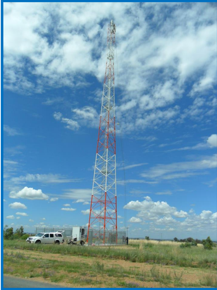
Plate 3: View of telecommunication mast
