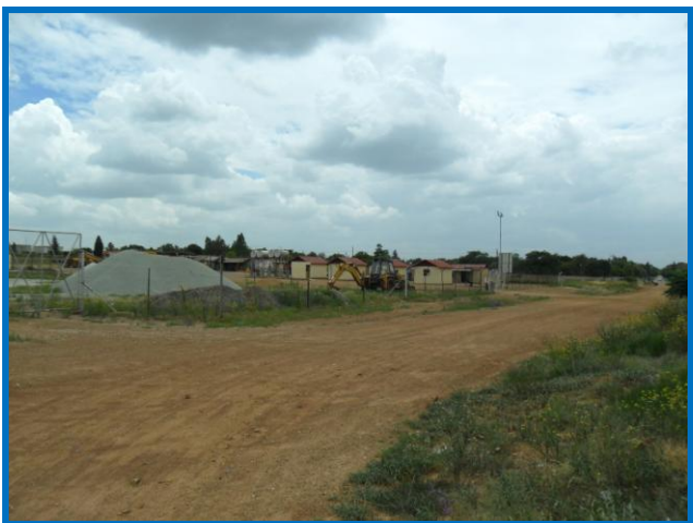
Plate 8: Public Works site
