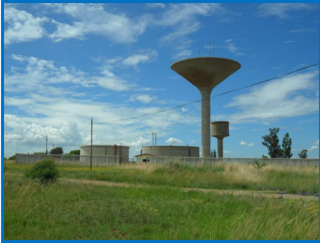
Plate 4: Ventersdorp Reservoir infrastructure
