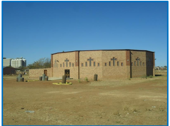
Plate 6: View of church facility adjacent to north-eastern corner of development area
