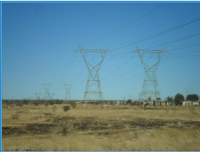
Plate 7: View of powerlines (direction south)
