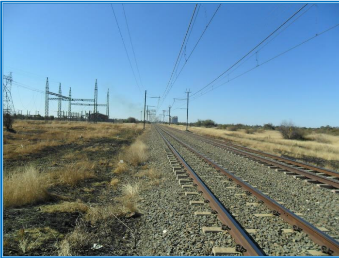
Plate 5: View of main railway line
