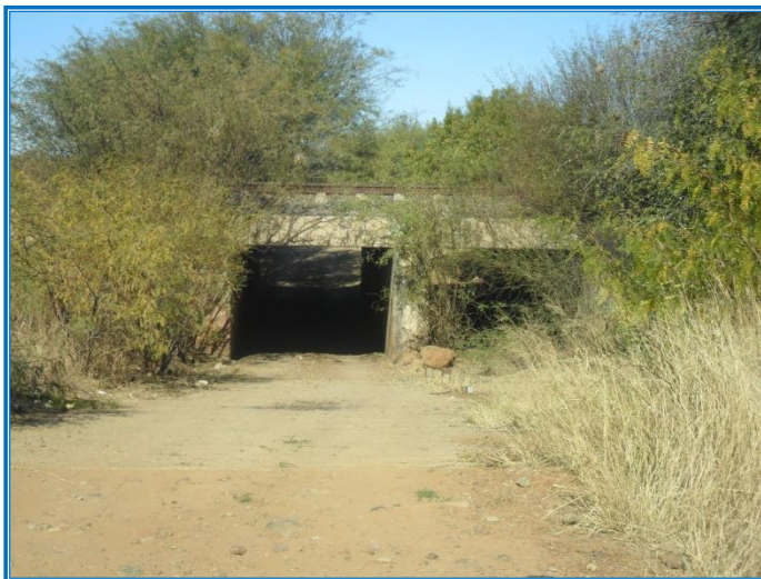
Plate 17: View of existing rail over road culvert crossing
