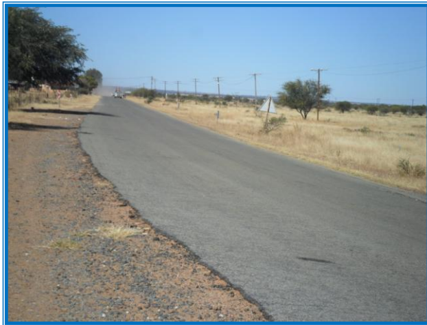
Plate 15: View of Road 462 (south)
