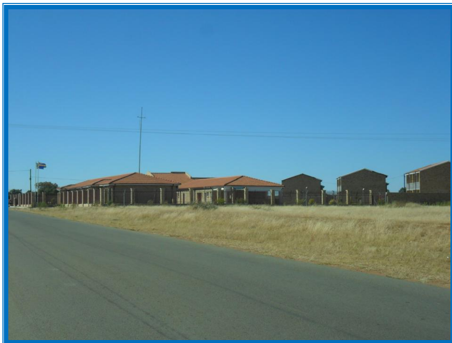
Plate 9: View of Amalia Community Safety Centre
