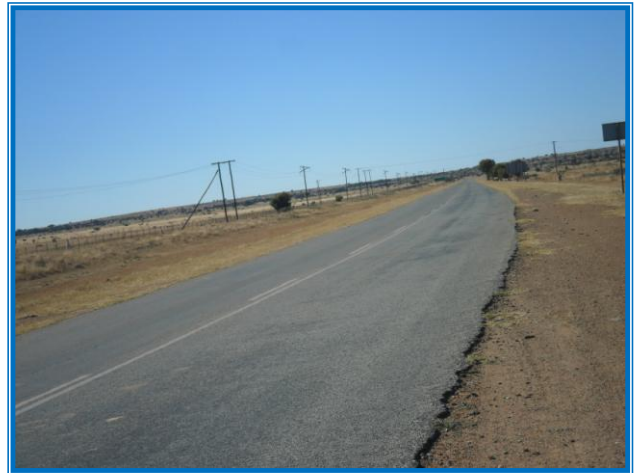
Plate 16: View of Road 462 (north)
