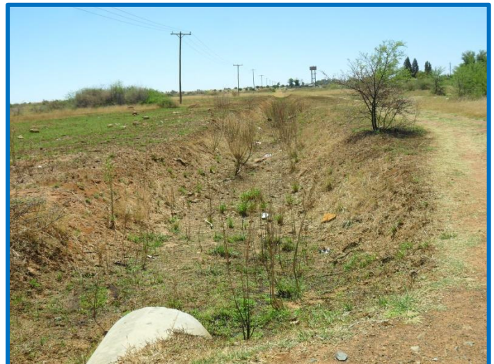
Plate 21: View of informal drainage channel (direction north)
