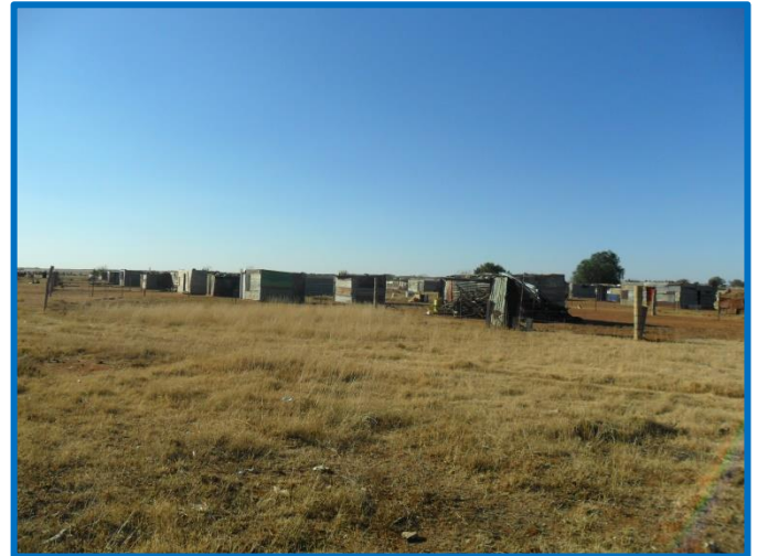
Plate 2: View of informal housing structures
