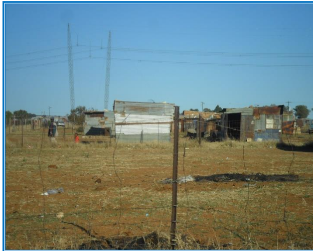
Plate 1: View of informal housing structures
