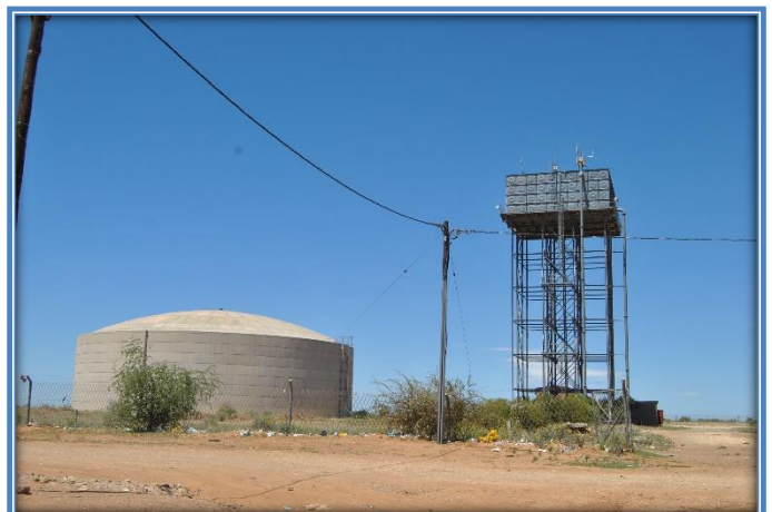
Plate 10: View of new ground- and elevated reservoir in Vryburg Extension 28
