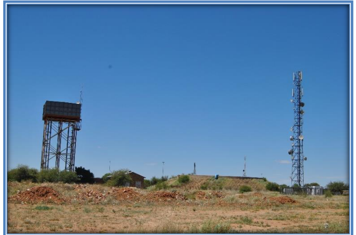
Plate 8: View of Huhudi elevated- and ground reservoirs
