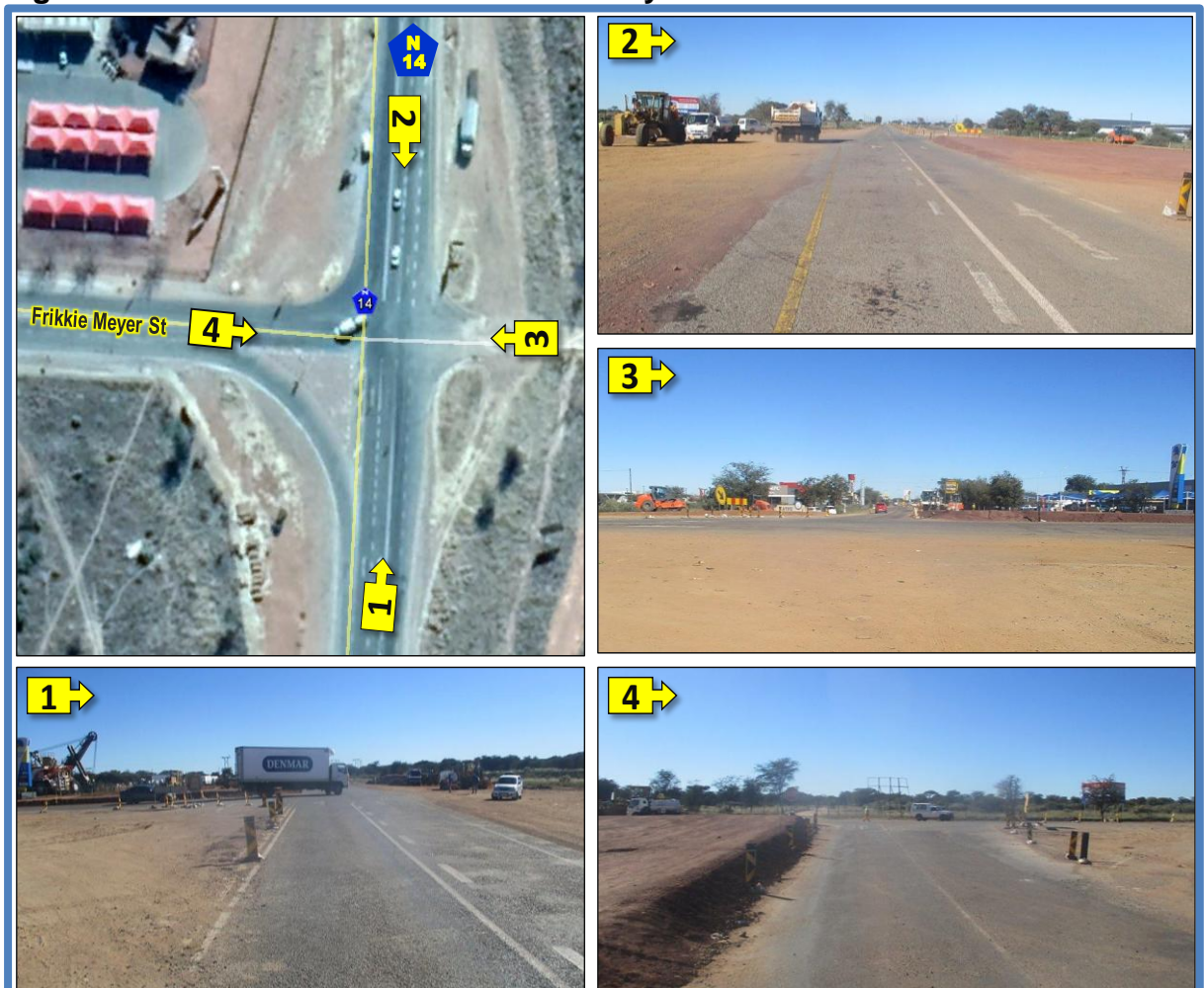
Figure 27: SANRAL Construction Underway
