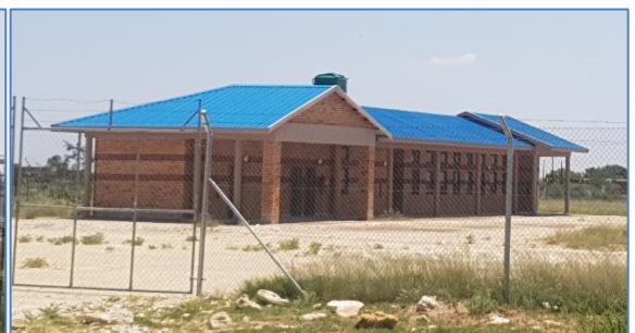
Photo 4: Churchill Traffic Offices
