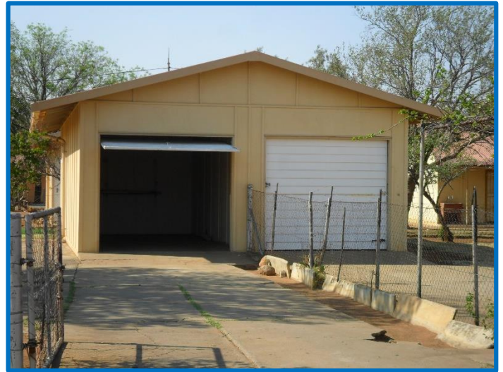
Plate 2: Existing outbuildings (garages)
