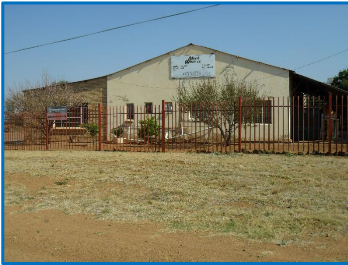
Plate 11: Existing commercial/business infrastructure on Erf 815 Wolmaransstad Extension 7
