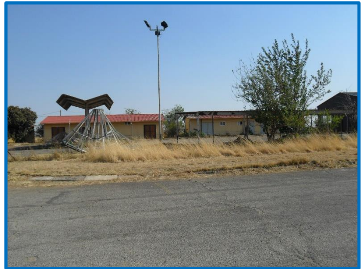
Plate 4: Dep Public Works and Roads workshops and storage areas
