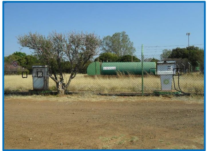
Plate 10: Existing diesel depot on Erf 814 Wolmaransstad Extension 7
