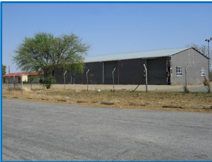
Plate 3: Dep Public Works and Roads workshops and storage areas
