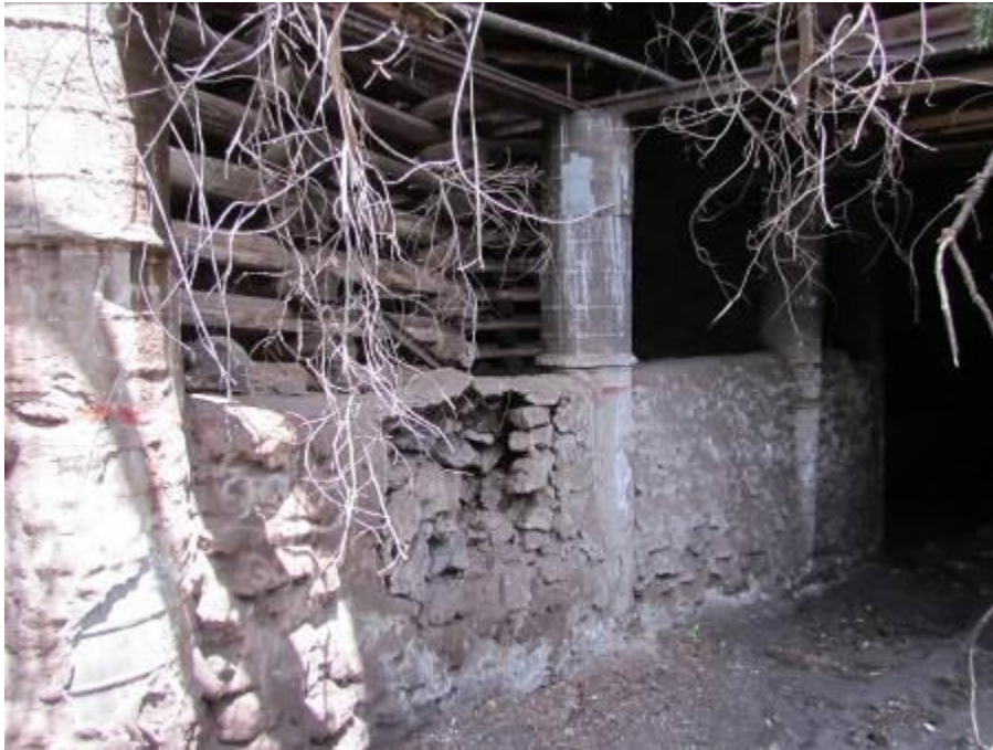
Figure 5: Retevment walls at historical mine entrance
