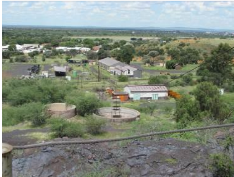
Figure 13: View of water reservoirs in the middle of the photograph
