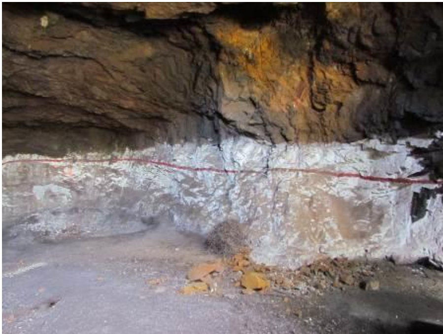
Figure 6: Historical mine shaft with a small rock fall
