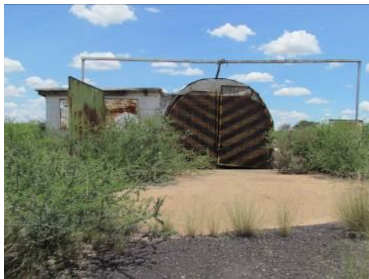
Figure 14: Surface structure of decline shaft
