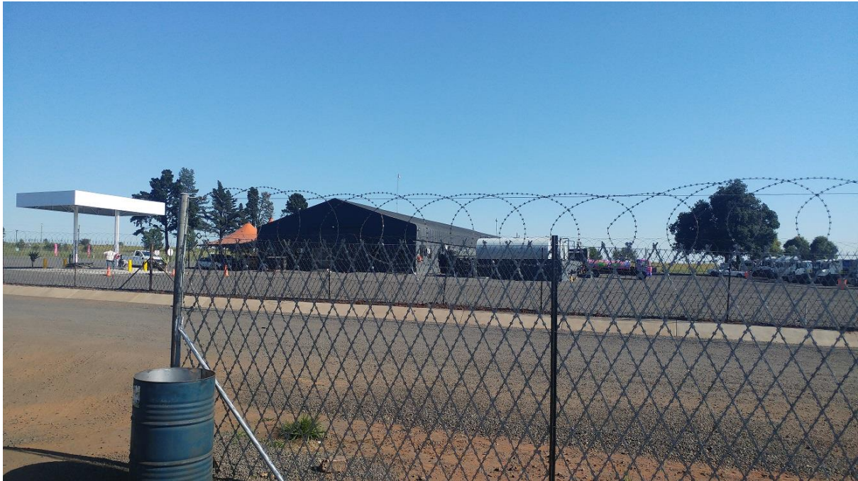
FIGURE 8: PROCESSING OR STORAGE BUILDING AT THE SURVEYED AREA.
