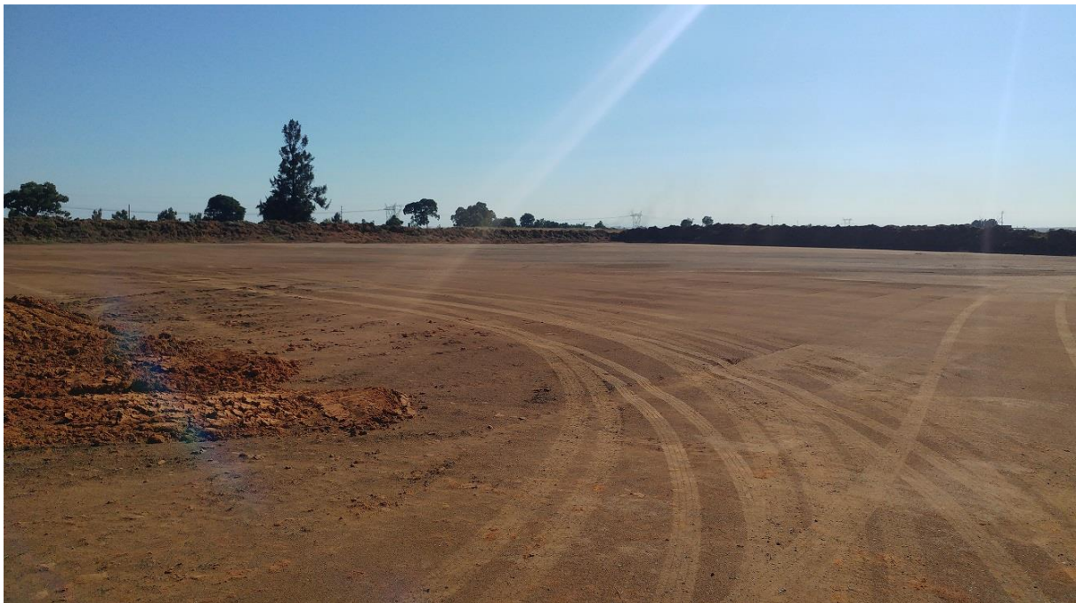
FIGURE 11: EARTHWORK ACTIVITIES IN THE SURVEYED AREA
