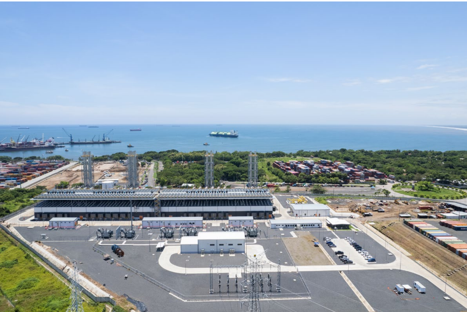
Figure 17: Aerial view of the 378 MW Acajutla Gas Engine Power plant fed directly from the 137,000m 3 FSRU BW Tatiana as seen in the distance.
