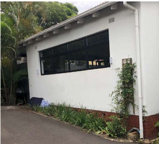
side views of ex. Dwelling showing new aluminium windows
