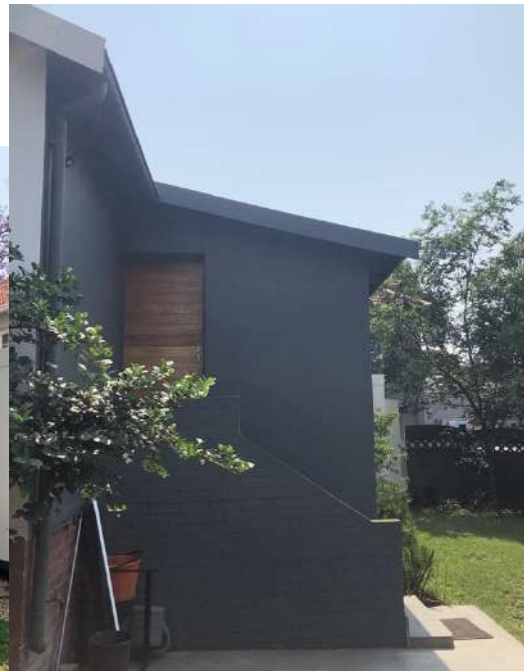
Side view of raised Study roof
