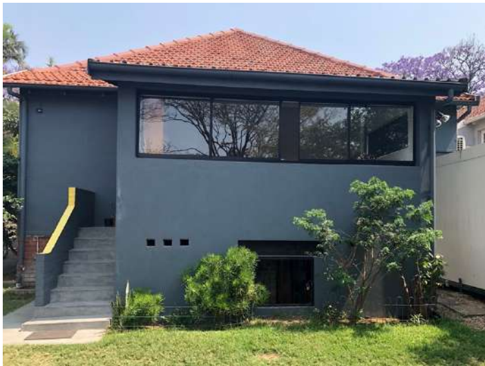
Back view showing new raised roof & new window
