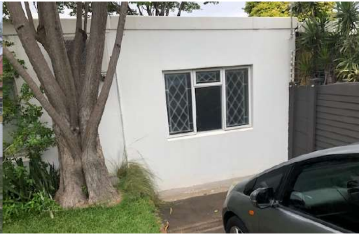
View of Garage converted into Ancillary unit
