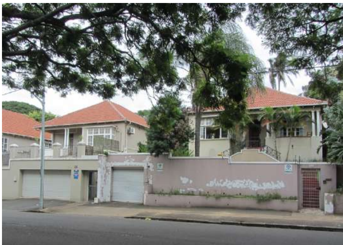
Street view of properties across the road
