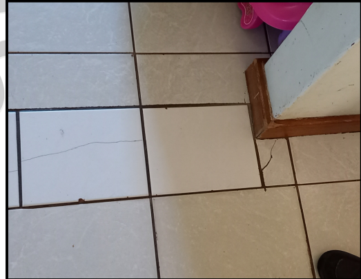
Cracks formed on floor.
