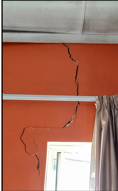
Cracks formed on masonry walls.
