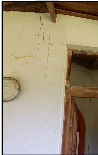
Cracks formed on masonry walls.
