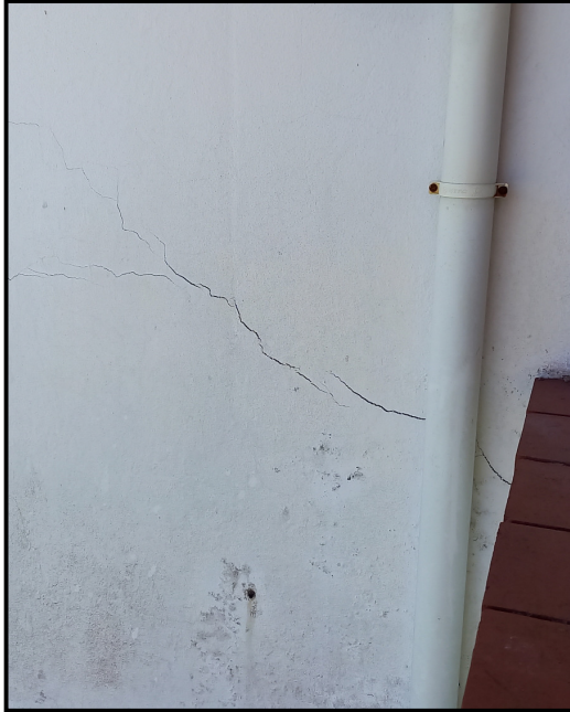
Cracks formed on masonry walls.
