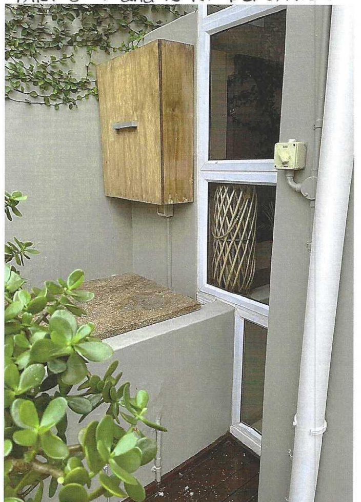
VIEW of new window - S.W. Elevation (enclosed verandah).
