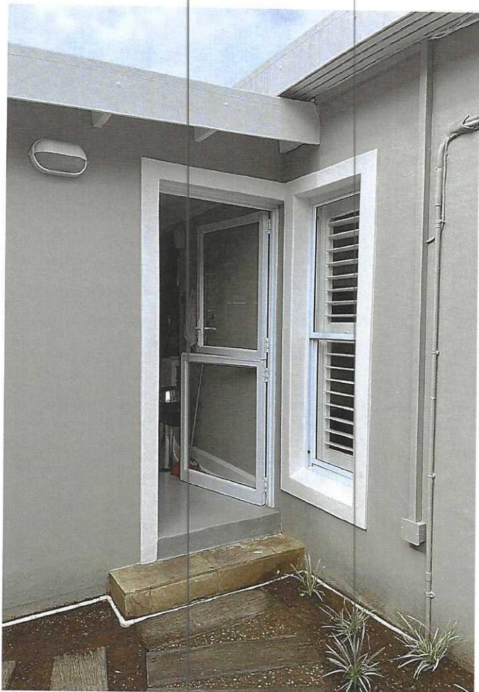
DOOR to existing scullery - N.W.
