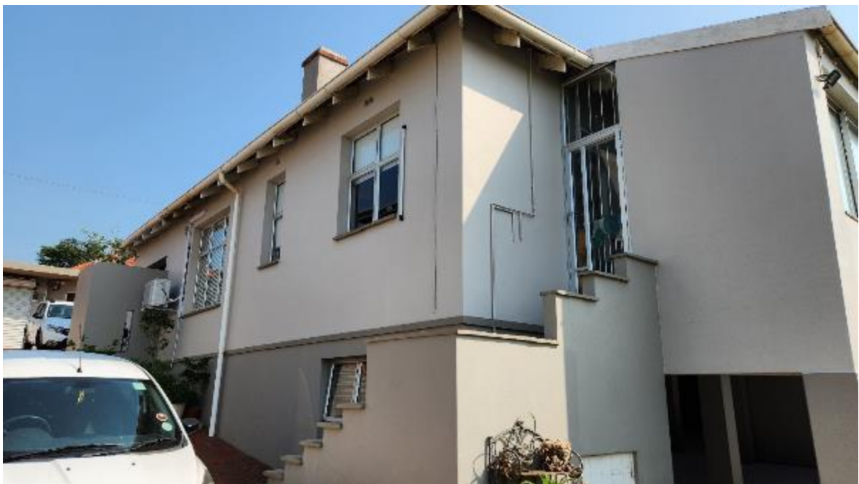
South-West Elevation - Internal
