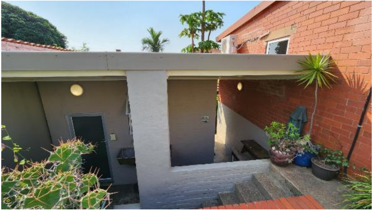
Outbuilding North-West Elevation
