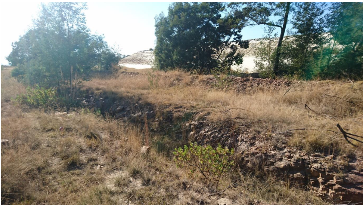
Figure 7-3: Berm located on the north-eastern side of the TSF
