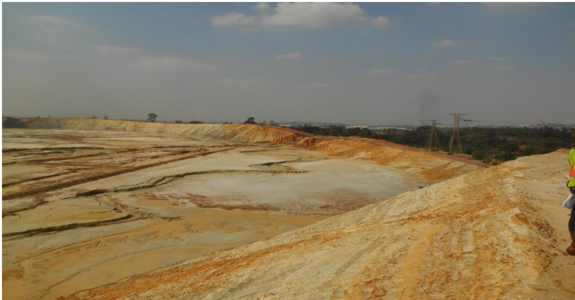
Figure 7-5: An example of the outer areas of a TSF acting as walls and containing dirty water runoff
