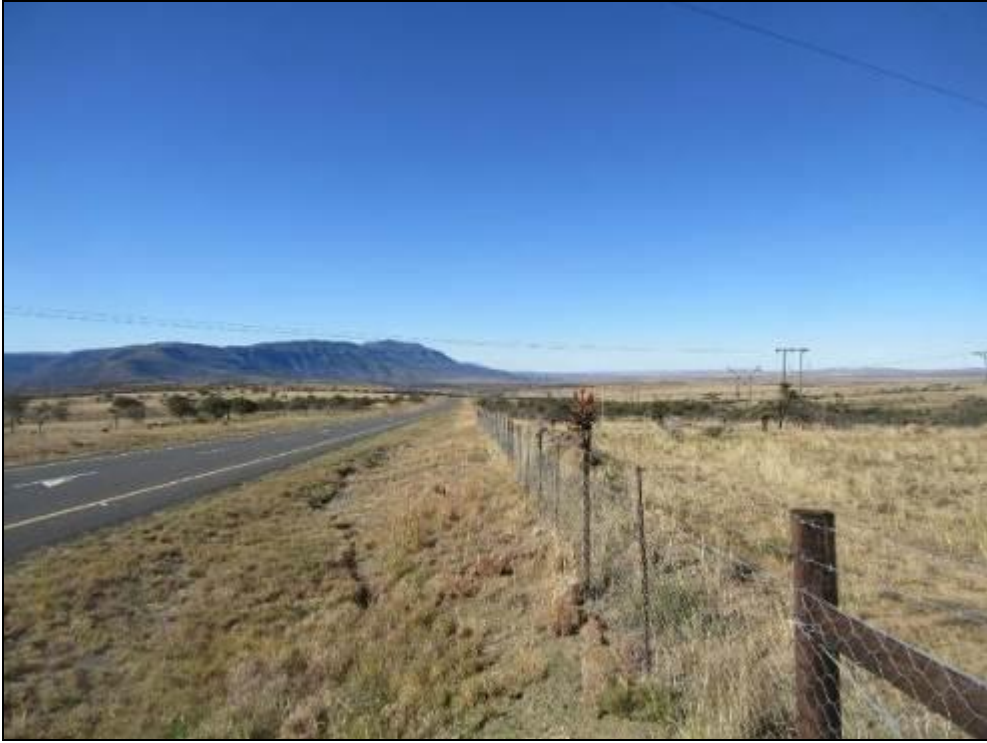
Photograph 3.4: Eskom 66 kV and 132 kV lines crossing the R63
