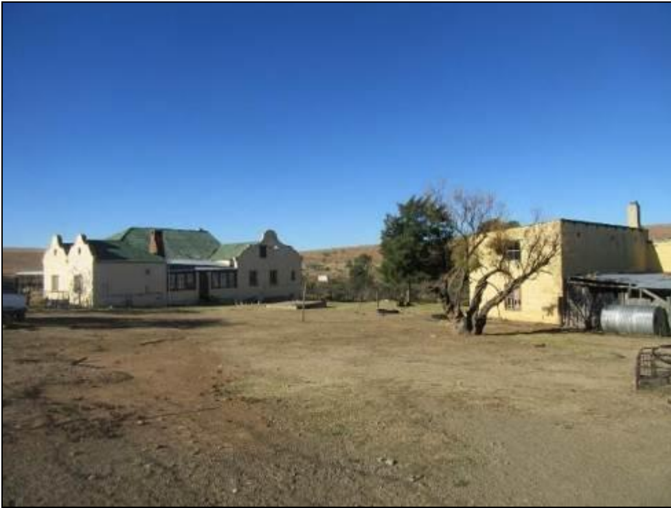
Photograph 3.14: House on Mulderskraal occupied by the son of the tenant, Mr Nelani. Mr Nelani resides in Somerset-East.
