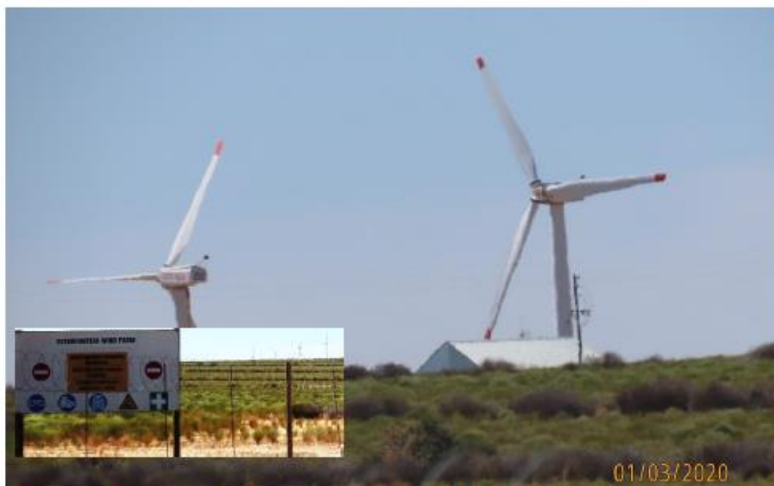
Figure 2: Red-tipped turbine-blades on turbines at the Ysterfontein wind farm north west of Clanwilliam in the Western Cape (S 32° 9'23.42" E 18°49'7.10"). While these mitigations are not used in the correct single-blade configuration used by the Norwegians, they set a precedent for turbine blades to be red-painted in South Africa © RE Simmons
