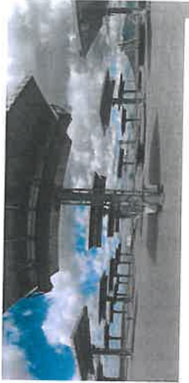
In storm: >28 mph. > 10 sec. Out of slow: <26 mph. >300 sec. Figure 6: Storm Slow position
