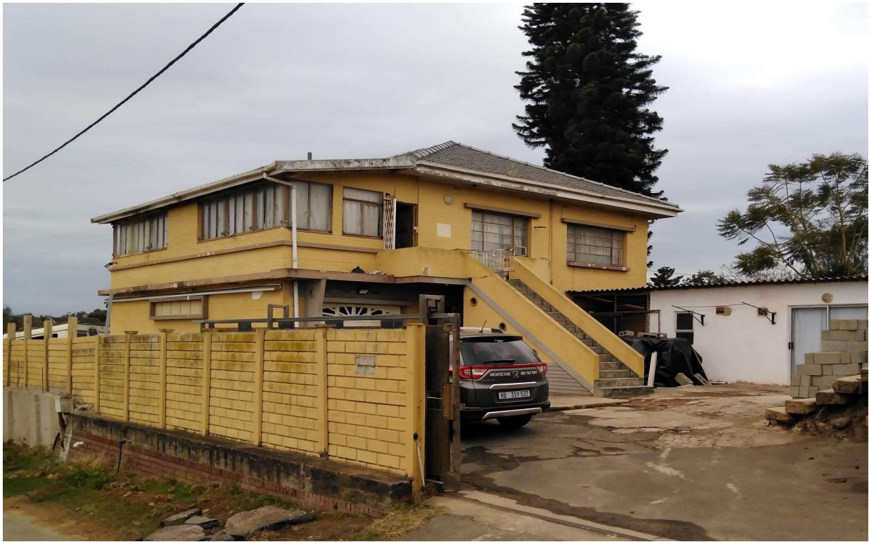
ROAD ELEVATION (DERING RD ) - EX DWELLING & NEW PRVI GYM - ILLEGAL BUILDING )
