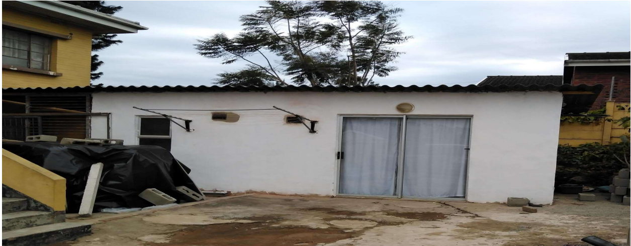
NEW PRIV GYM = W. ELEVATION (ILLEGAL BUILDING - OLD ROOF IN)
