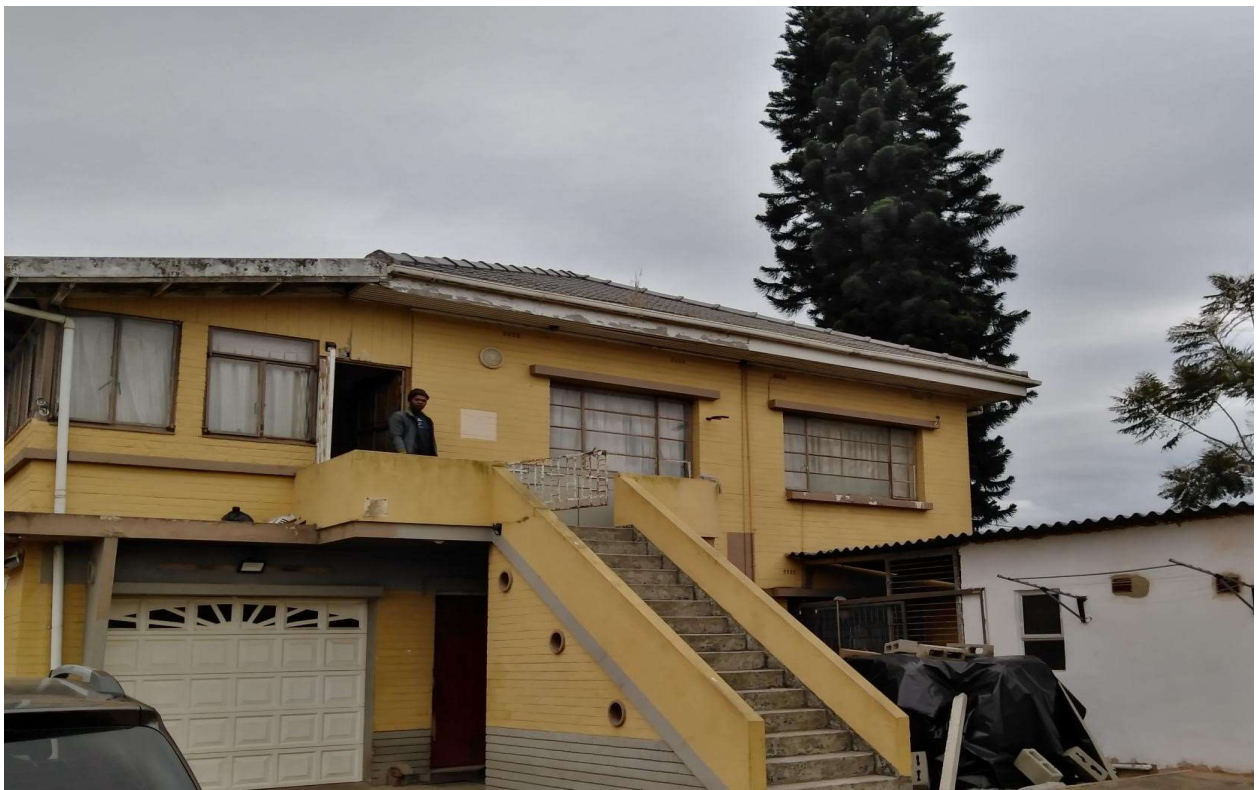
EX DWELLING & NEW GYM (ILLEGAL BUILDING - OLD ROOF IN )
