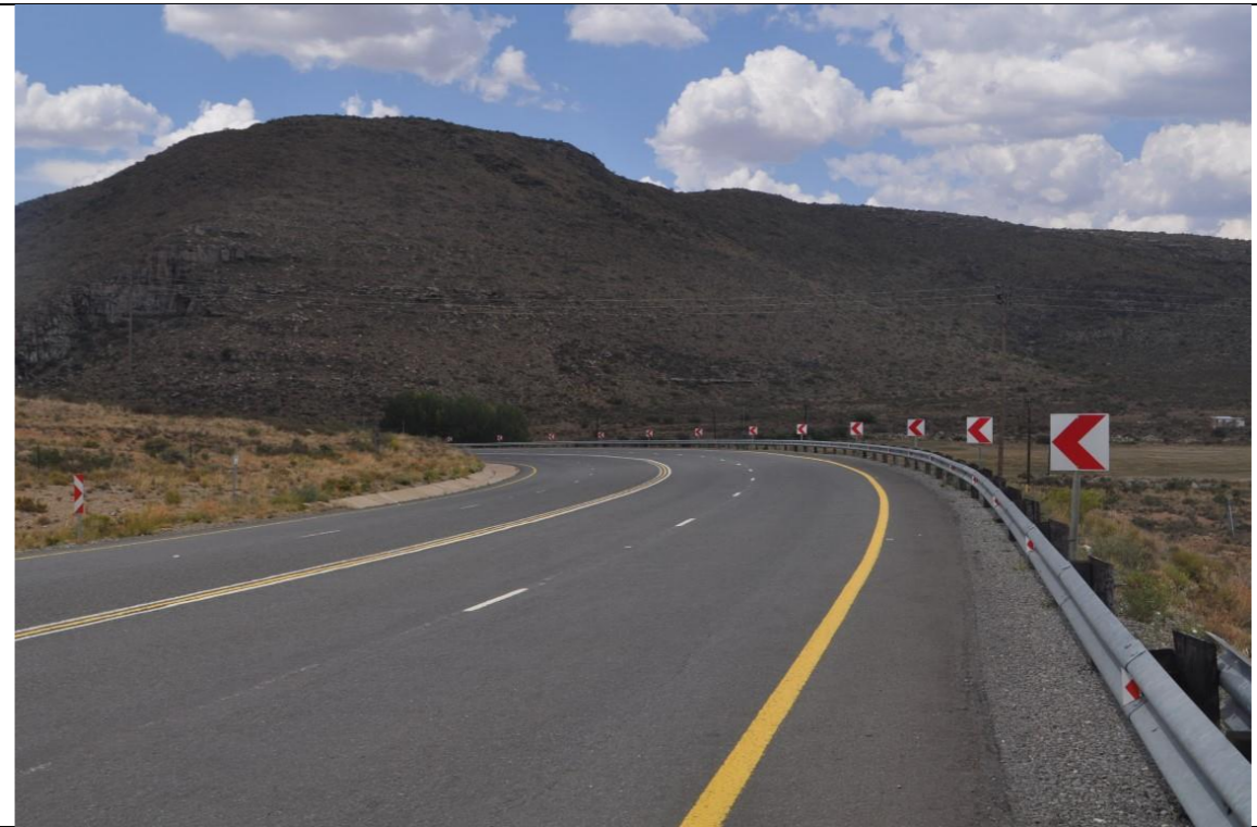
Right Approach (vehicles approaching at high speed on super elevation)
