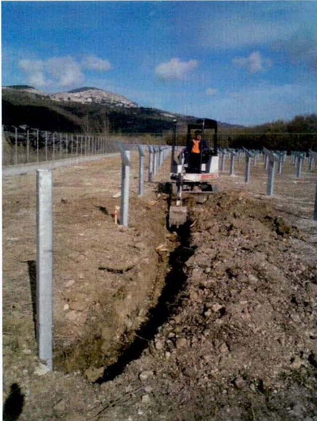
Figure 2.6: Trenching for underground cables for the PV panels
