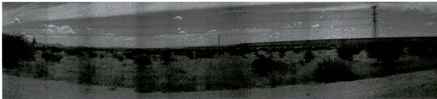
View 9 looking north from internal road towards existing tailings facility
