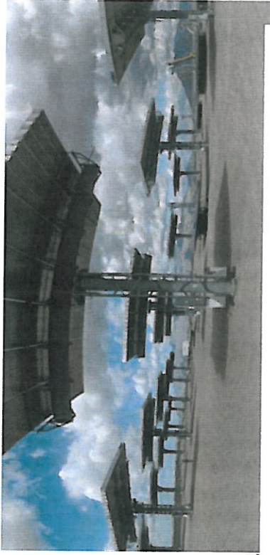
In stow: >28 mph, > 10 sec. Out of stow : <26 mph, >300 sec. Figure 6: Storm Stow position
