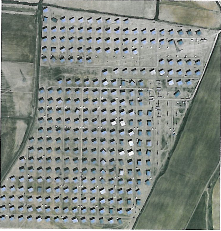
Figure 3: Typical Solar Farm layout
