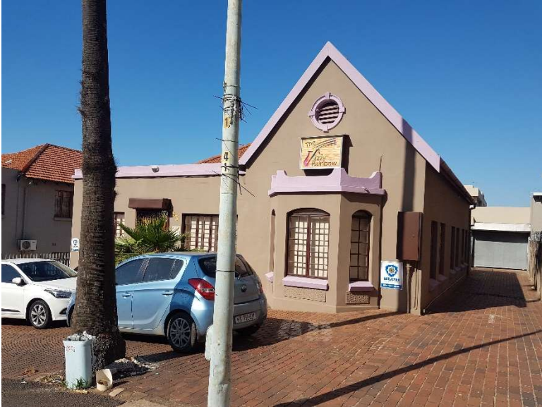
NORTH ELEVATION – VIEW FROM GOBLE ROAD
