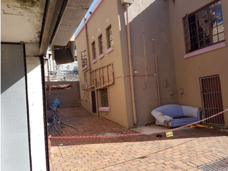
SOUTH EAST ELEVATION – FROM REAR
