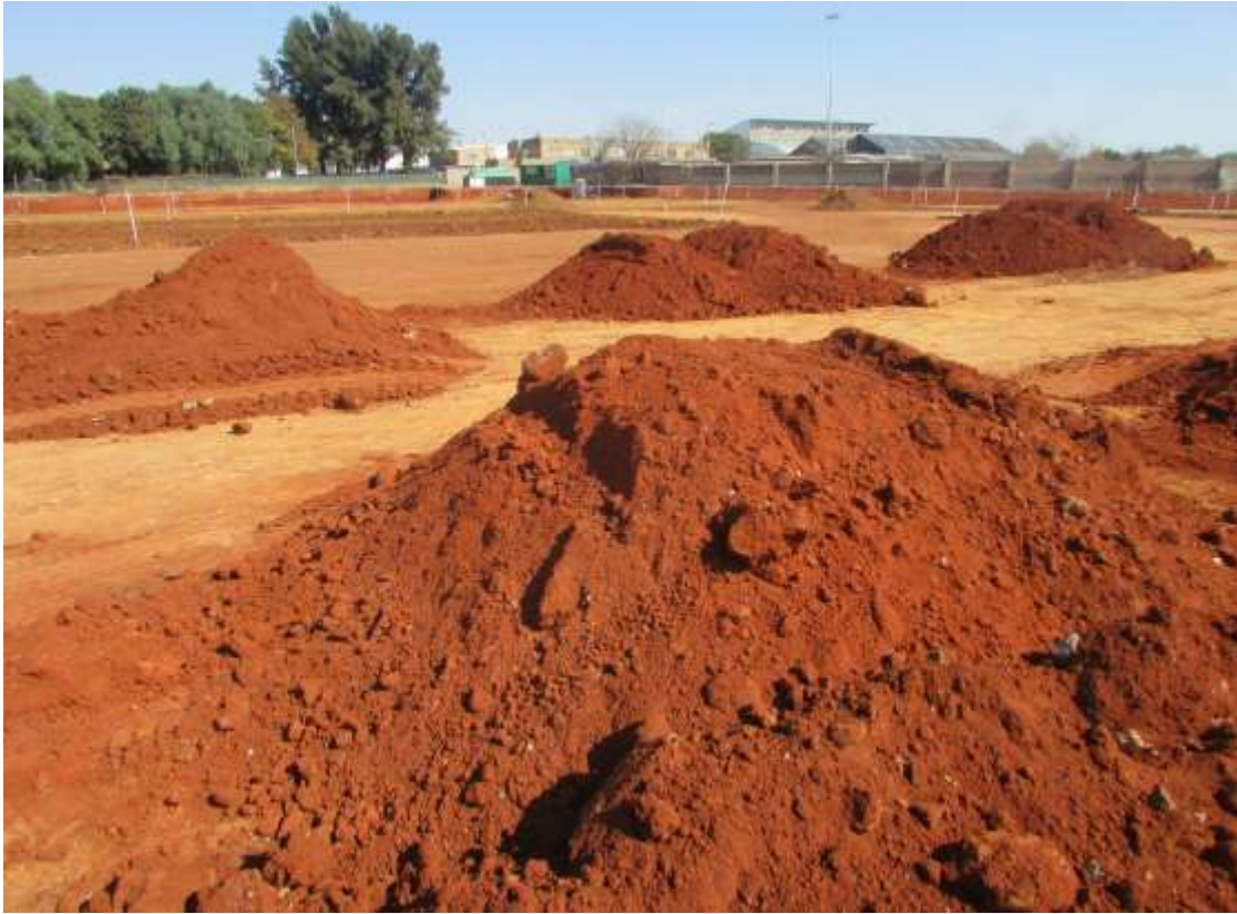
Figure 1: Spoil heaps where the human remains were initially identified by the Contractor.
