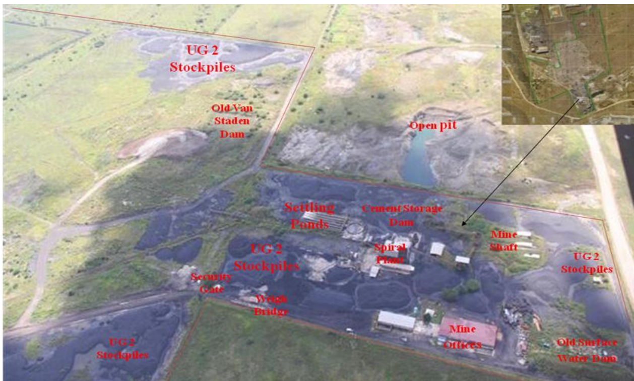
Figure 4(b): Photo showing the Mine Plant Layout of MA-1.
