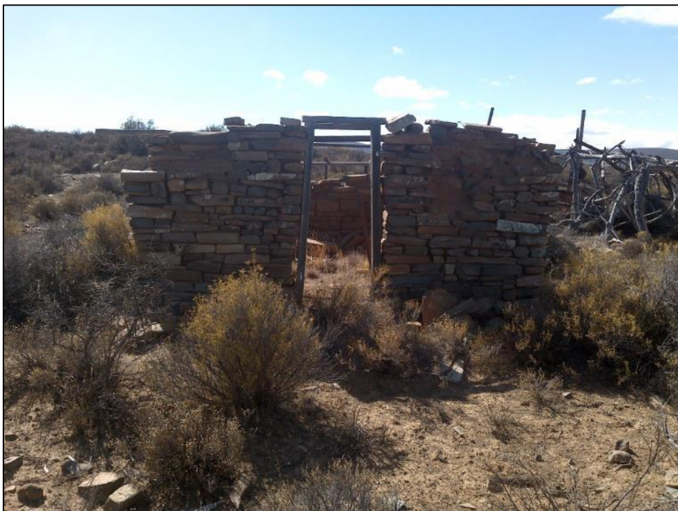
Figure 37: Close-up view of the stone walling cottage (BV_SW4) facing east.
