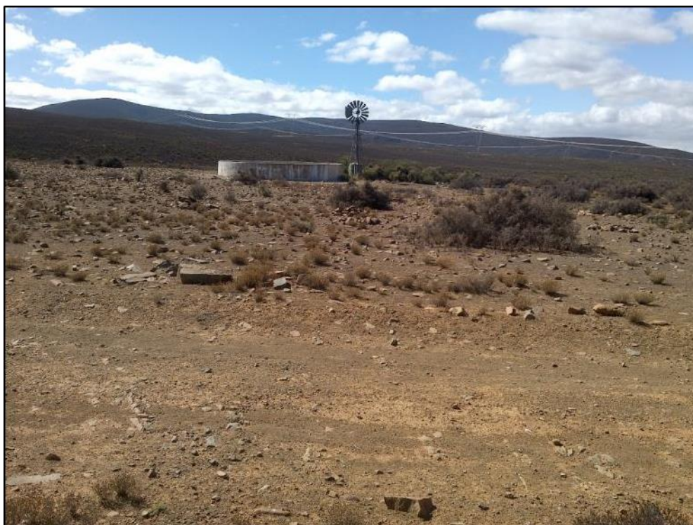
Figure 41: View of the reservoir (BV_BE4) facing east.
