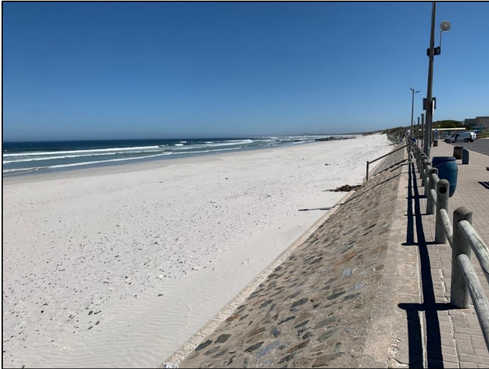
Figure 8. Seawall to the south of the concrete pathway at “Alternative 1”.
