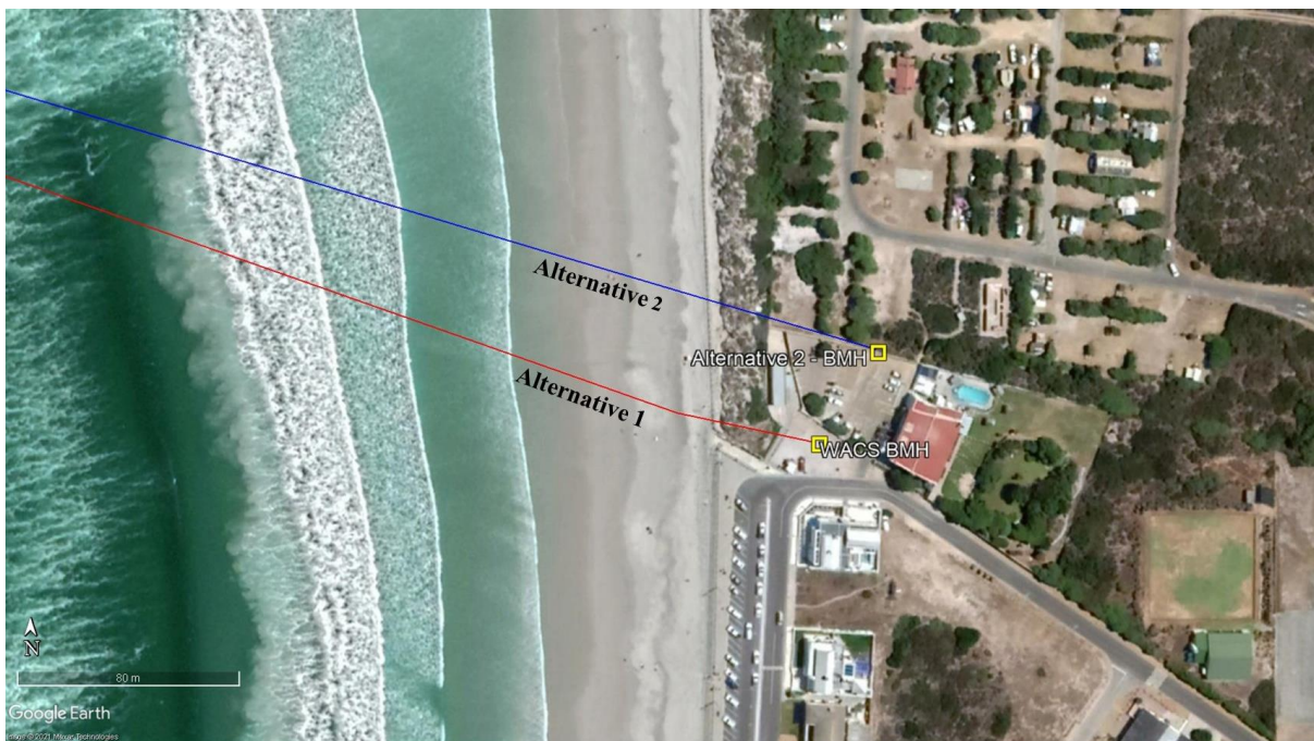
Figure 2. Image of site of cable landing at Yzerfontein, showing two minor variations or alternative routes.
