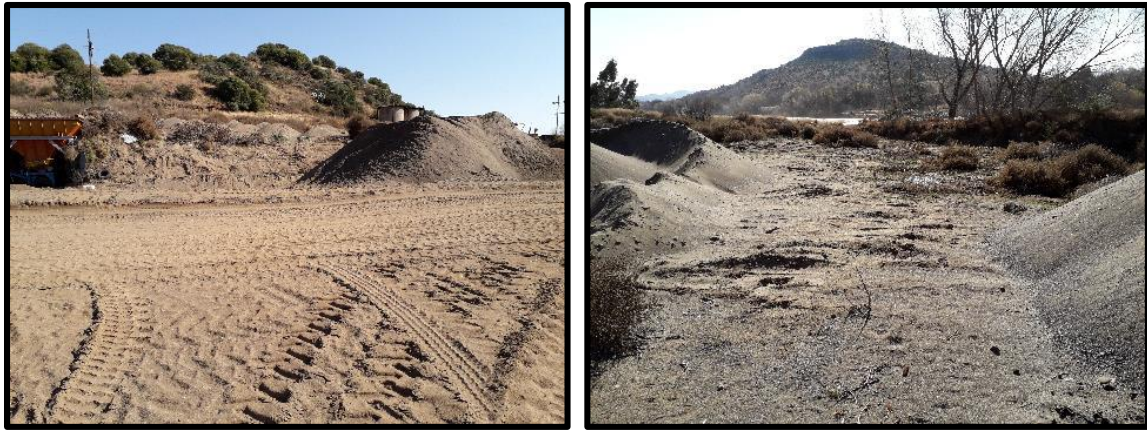
Figure 1: Photographs showing the proposed stockpile area that has been altered by the previous sand mining activities.
