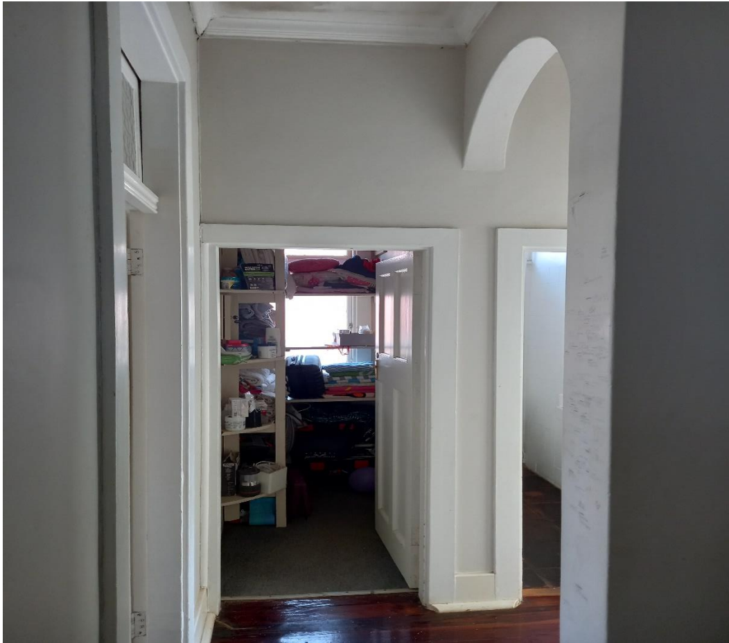
DOOR OPENING TO NEW BATHROOM FROM PASSAGE
