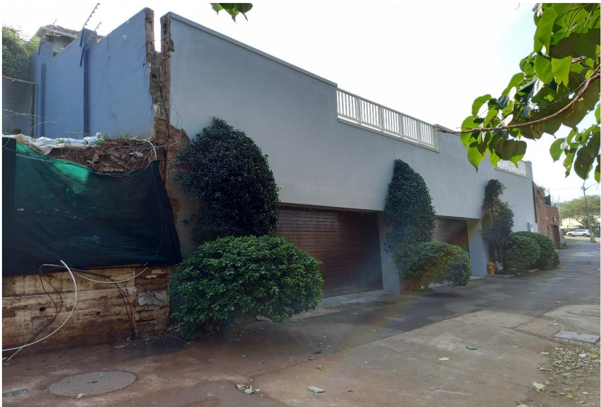
ADJACENT NEIGHBOUR RIGHT HAND SIDE
