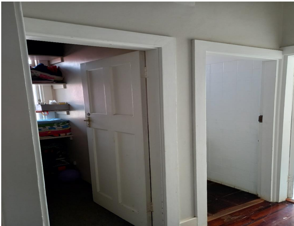
RIGHT HAND SIDE DOOR TO BE BRICKED UP
