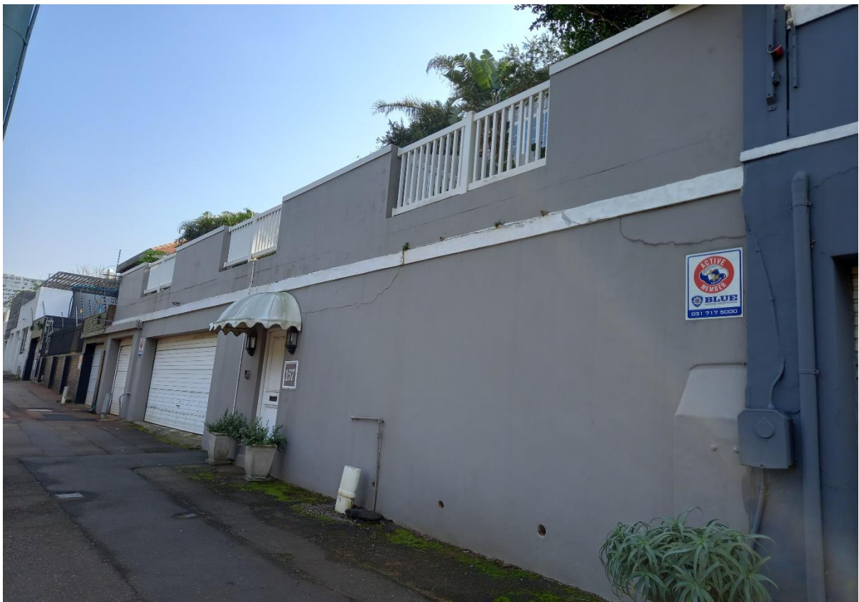
ADJACENT NEIGHBOUR LEFT HAND SIDE ROAD FRONTAGE
