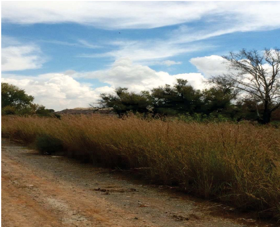
Figure 4-2: Photo 1 taken from an easterly direction. A view of the proposed pipeline route extending from Grootvlei Shaft 3 to existing Grootvlei 6/L/16 site
