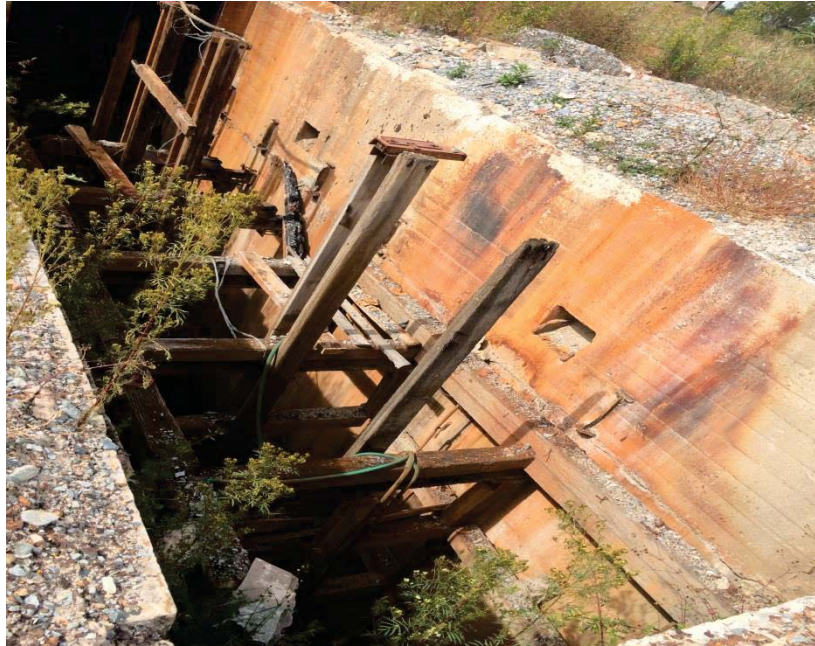
Figure 6-12: Grootvlei No. 3 Shaft
