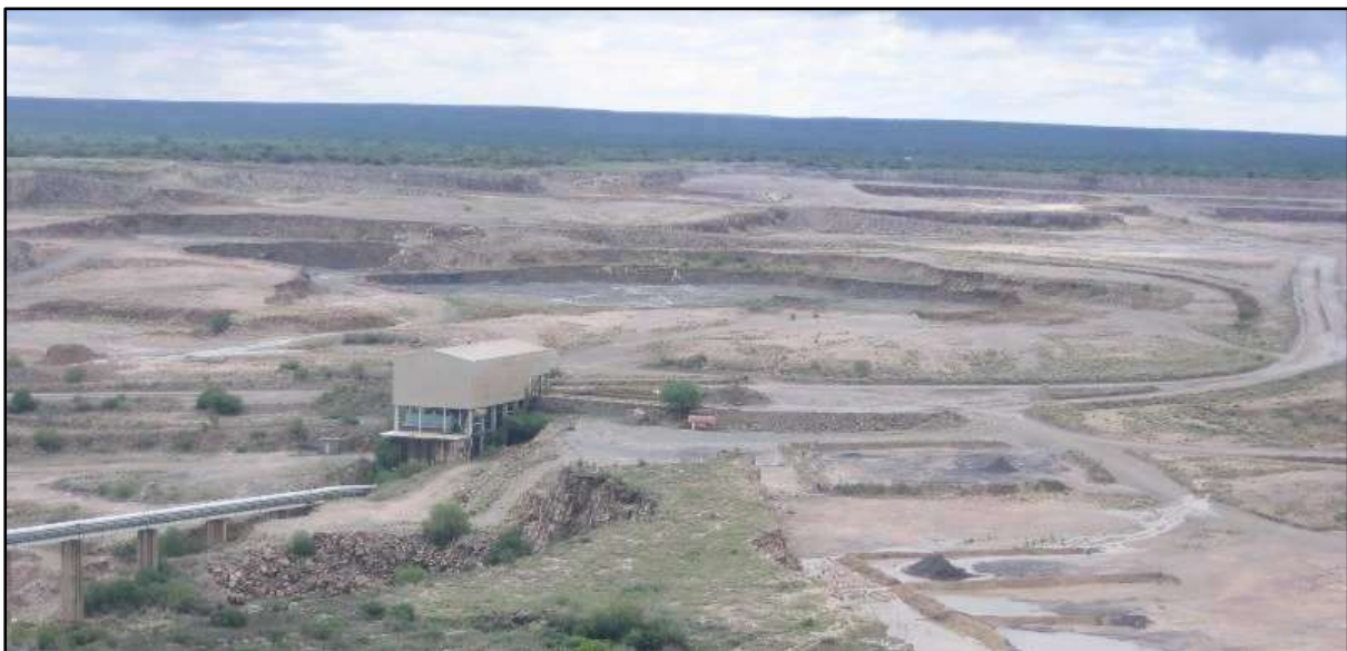
Figure 13: Crusher for materials less than 750 mm
