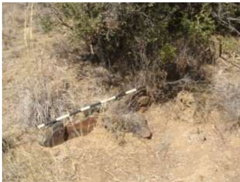
Figure 15: More stone walling near the water reservoir. This is the foundation walls of a possible hut.
