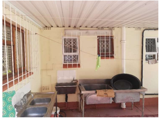
Image 6 Above: Main Dwelling Rear elevation
