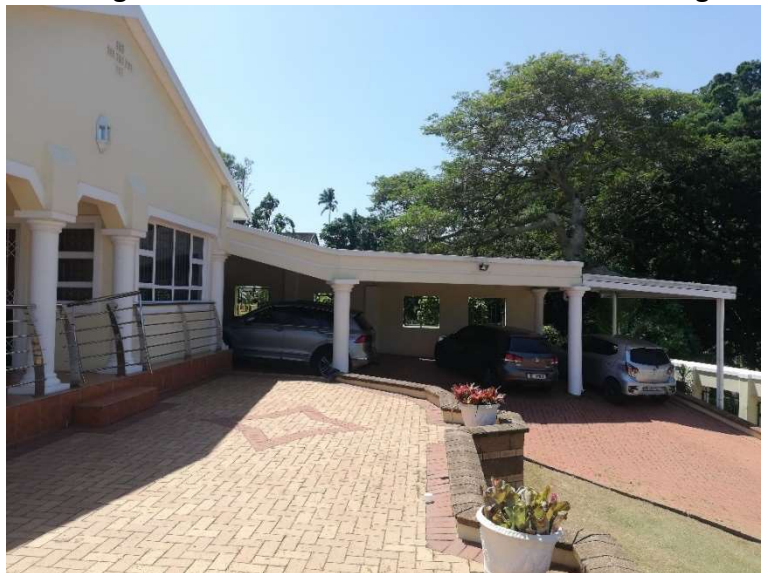
Image 2 Above: View from Main Dwelling looking at new covered parking
