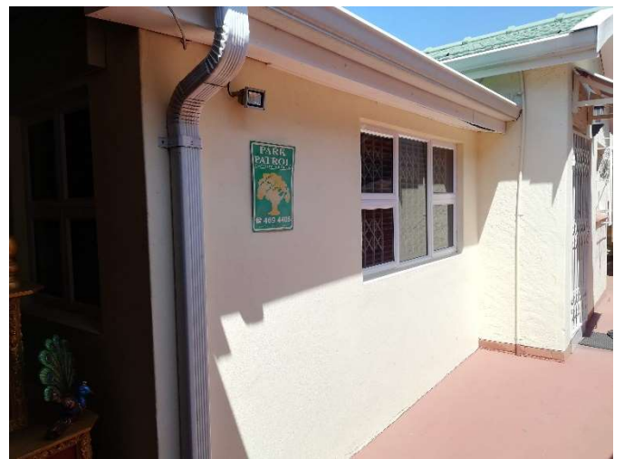
Image 8 Above: Main Dwelling Rear elevation
