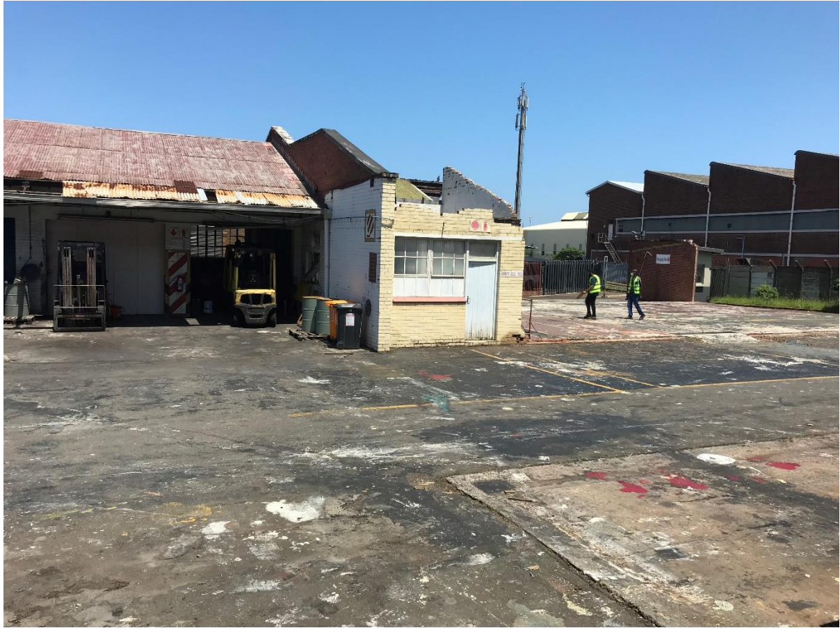
Figure 4). Image illustrates the region of the already demolished garage.
