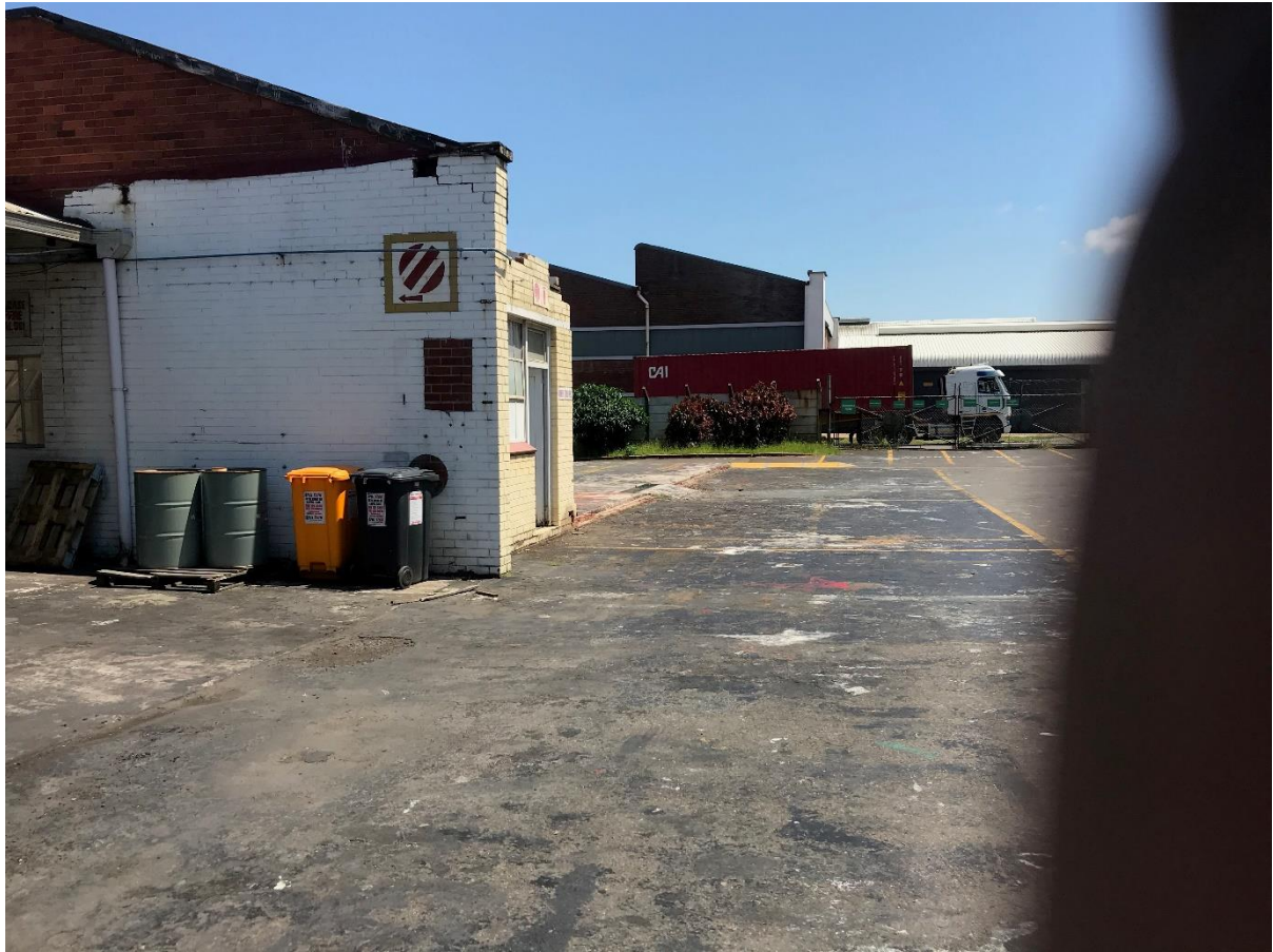
Figure 6). Image illustrates the region of the already demolished garage,
