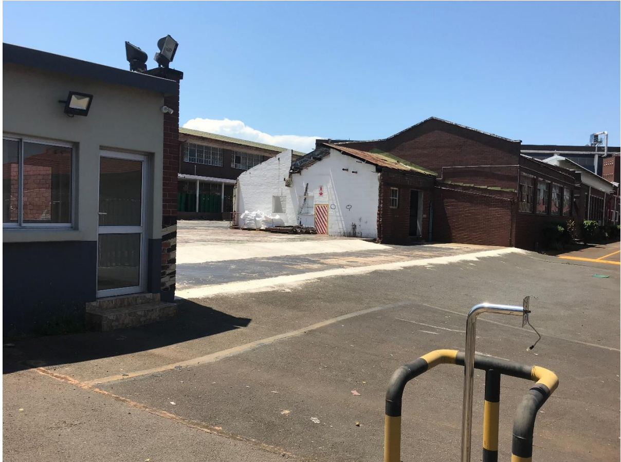
Figure 3). Image illustrates the region of the already demolished garage.
