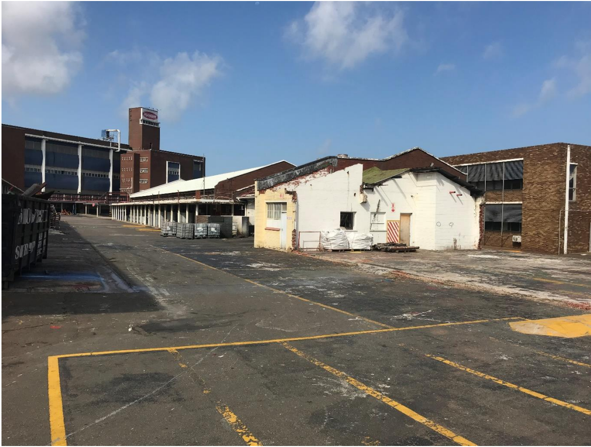
Figure 1). Image illustrates the region of the already demolished garage.
