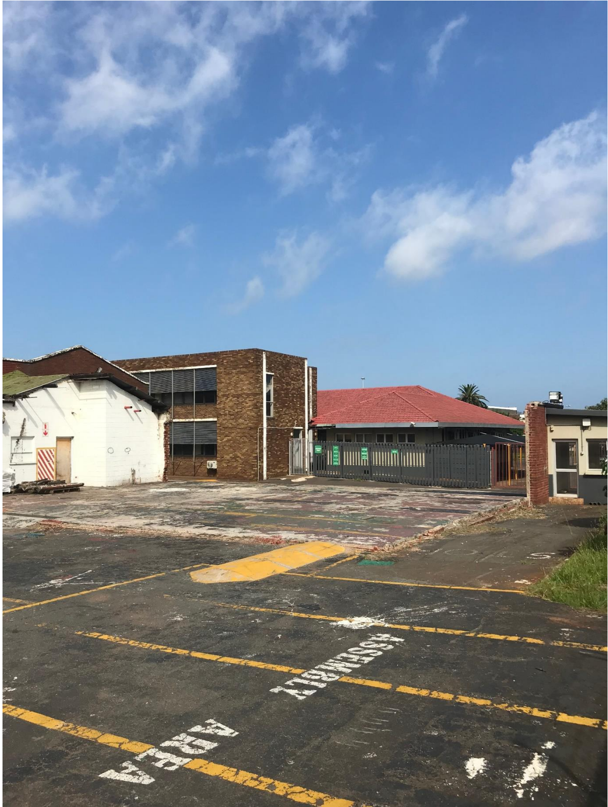
Figure 5). Image illustrates the region of the already demolished garage.
