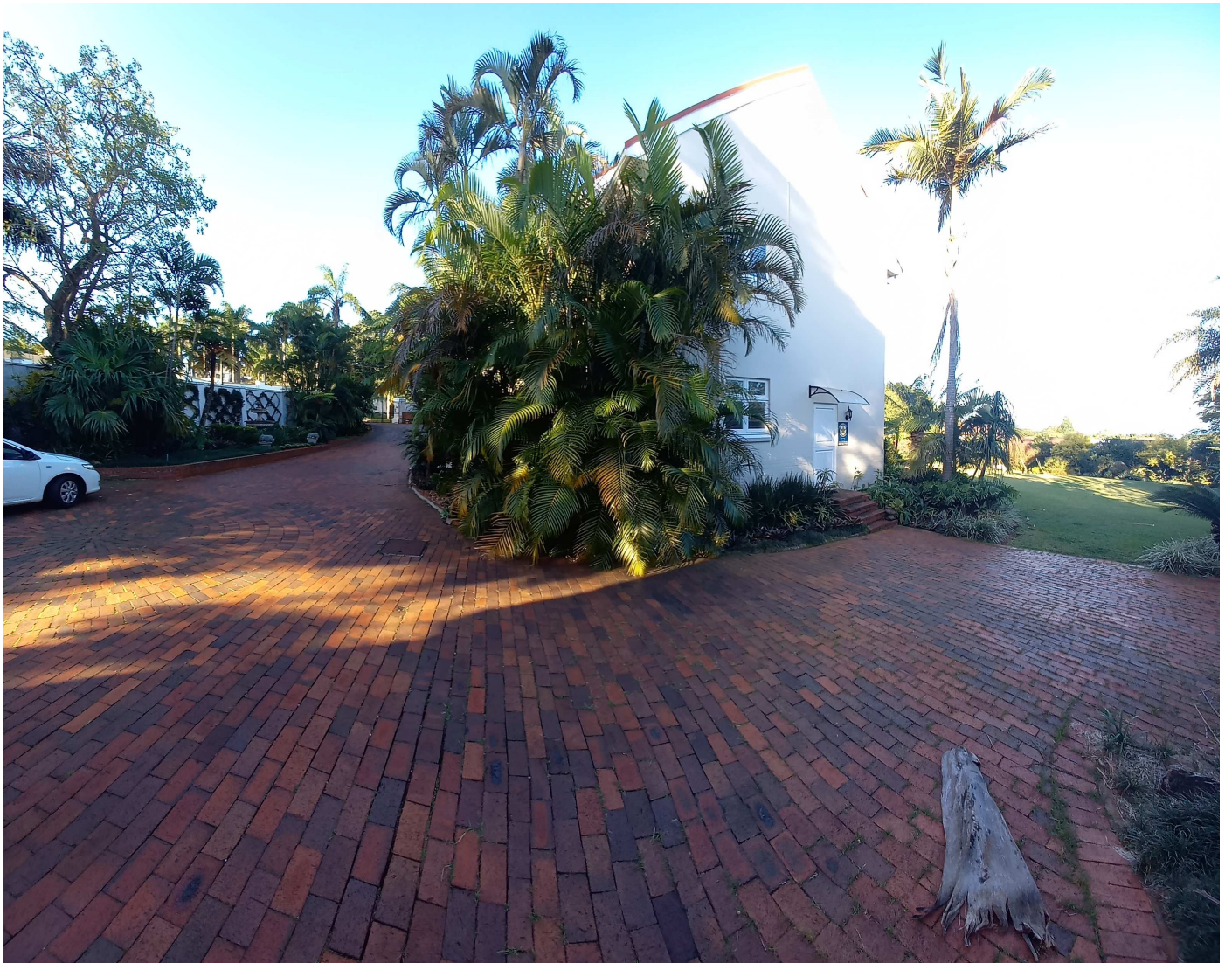
IMAGE ABOVE: South West Elevation of exg. House.
