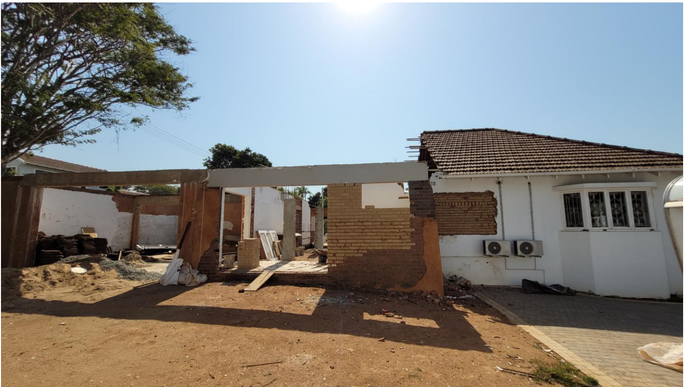
IMAGE ABOVE: Southwest Elevation of existing House.
