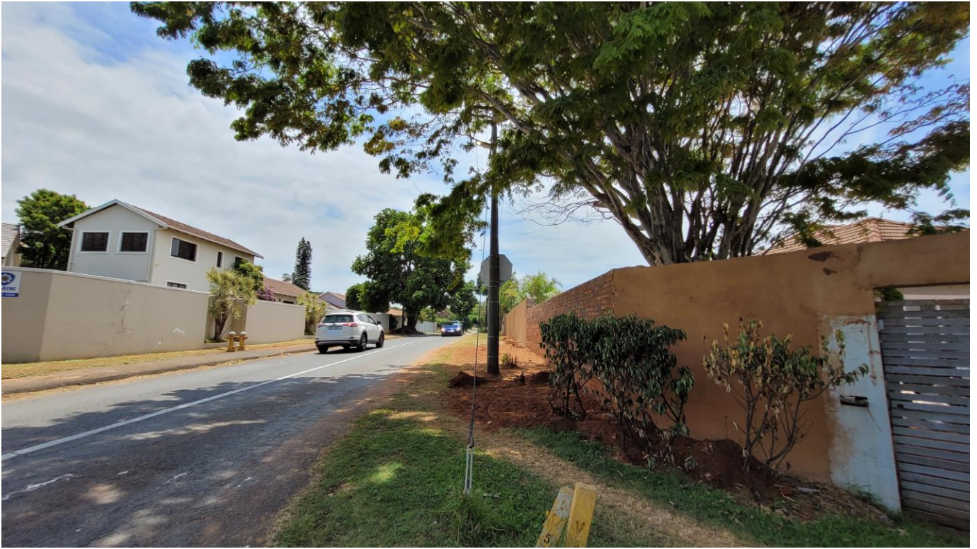
IMAGE ABOVE: Northwest street view of exg road and boundary wall.
